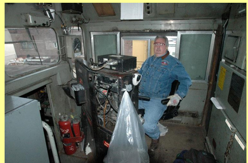
Illinois Division Engineer Don Scott at Sterling, IL on 02/09/06.
